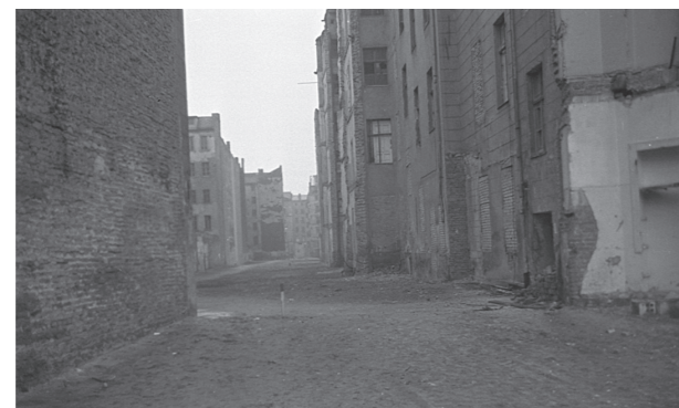
D 428: Torn down rear buildings and side wings on Bernauer Strasse, around 1965
