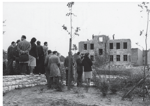
A 305: First demolition of a building at the border
